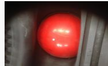
Bungs in casing to stop ingress
